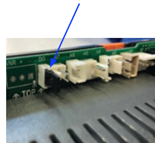
Jumper after installation
